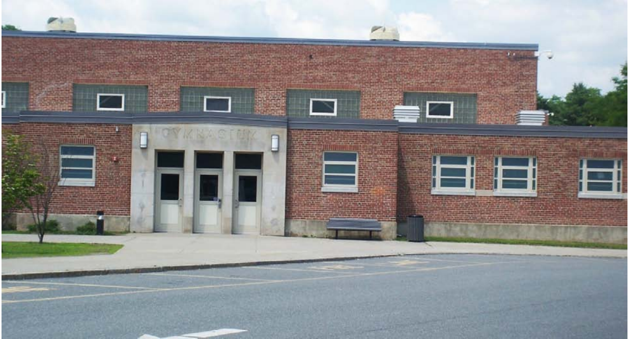
The entrance to the gymnasium is in the same place
